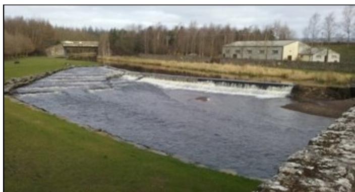
Fish-friendly rock ramp at Castletown Weir, Co. Laois
