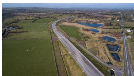
Fig 6.2. Aerial photo of compensatory habitat provided by the N4 road realignment project
