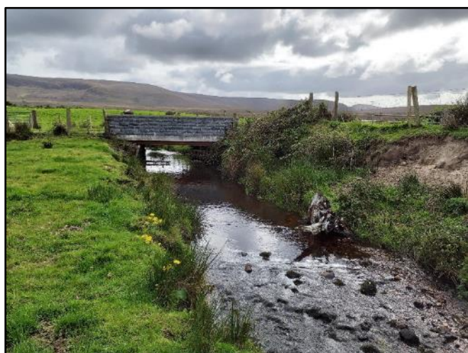
Leanrevagh West at Milltown Field (Site 8)
