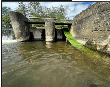
Photographs 1-3. Elvers trying to negotiate the vertical face at Cappogue Weir (L), construction (C) & installed elver ramp (R).
