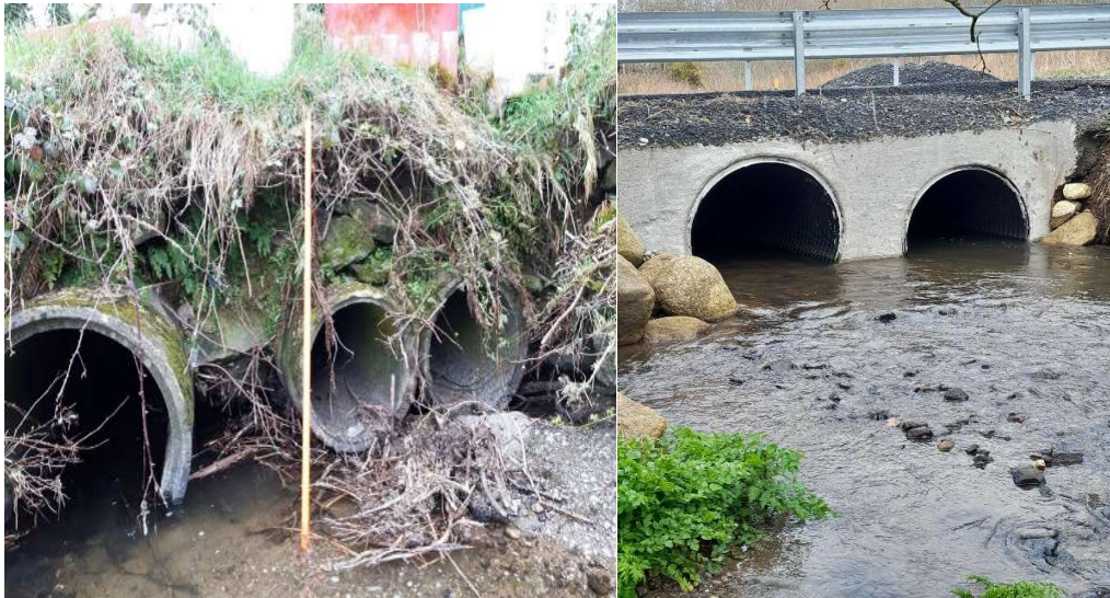
Figure XX Bridge before and after repair works
