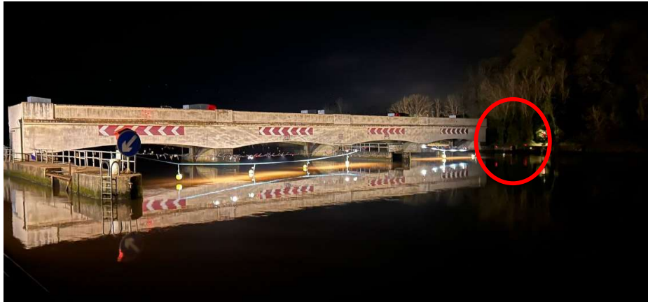
Figure 5-18 Photograph of deflection light array in operation with nets 1-3 lit and net 4 (circled) in darkness.
