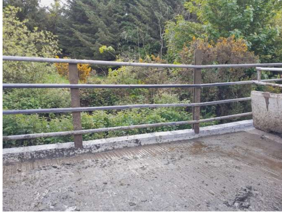
Figure XX Concrete berm to prevent run-off from yard (Arrigle Catchment)
