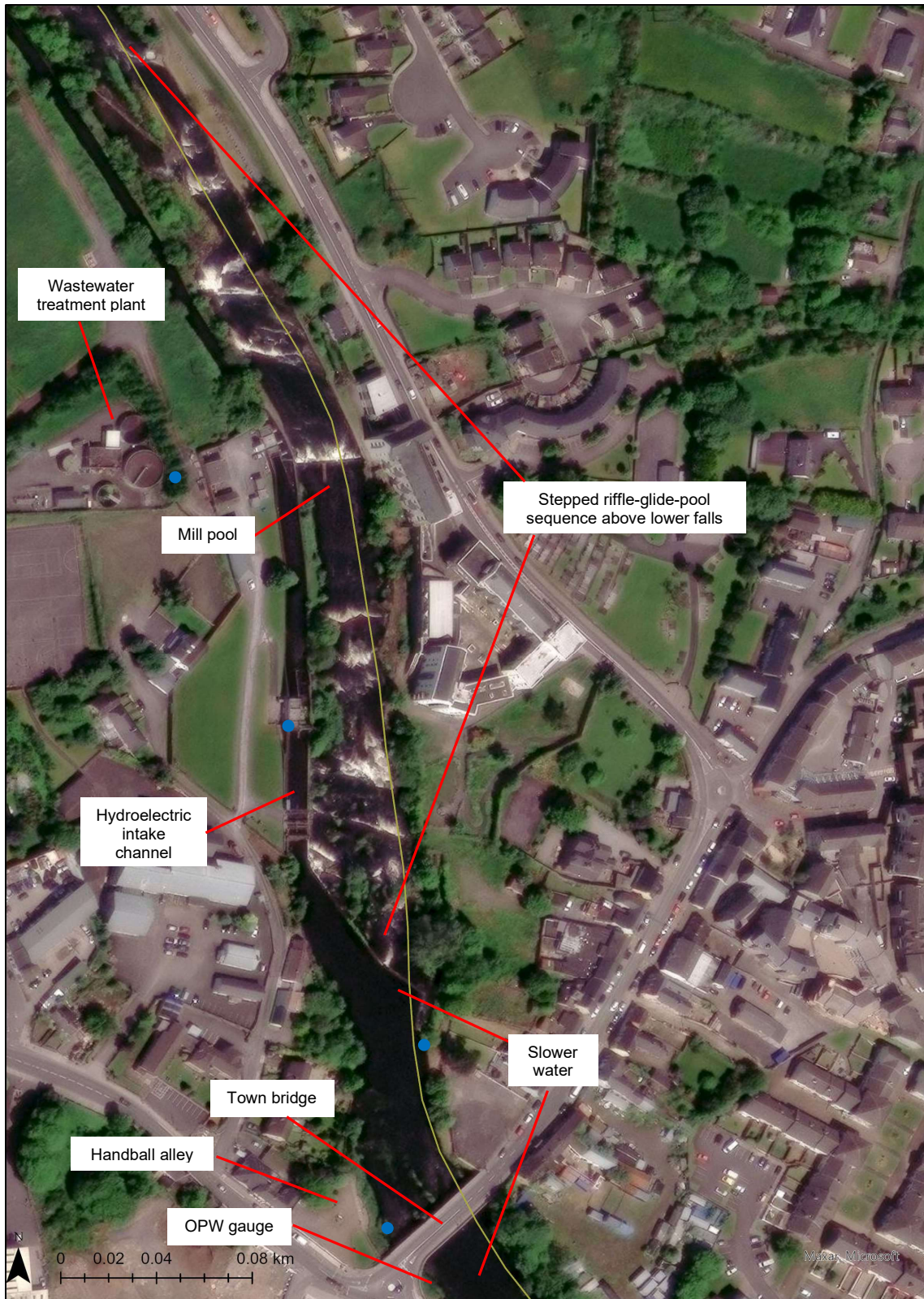
Figure 3b Satellite view of section of Lower Ballisodare river from above the lower falls to Ballisodare town bridge showing series of stepped riffle-glide-pool reaches above lower Ballisodare falls. Blue dots = storm water outflow points (Source: Esri, Maxar, Earthstar Geographics, and the GIS User Community).
