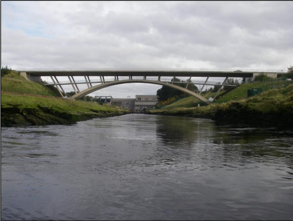
Plate 3.4. Cathaleen's Fall hydro generation power station on the Erne Estuary in the NWRBD.
