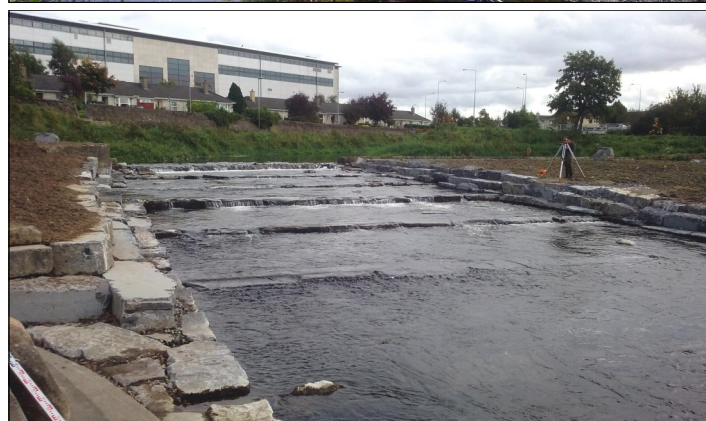
Top: survey at Askeaton Weir. Bottom: mitigation works at Hanover Weir.
