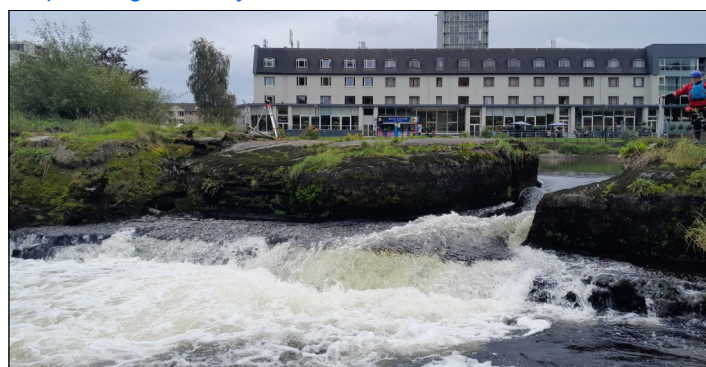
Barrier survey at Waterworks Weir on the River Lee
