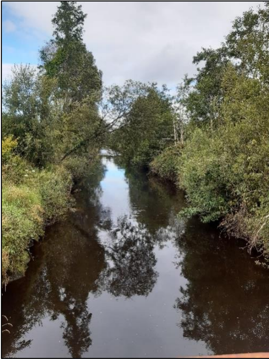
Plate 2. OPW drained section of the County River
