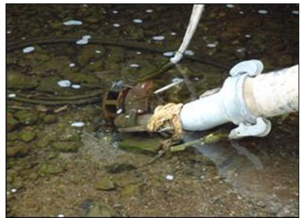
Continuous abstraction using submersible pump. No screening in place to prevent the entry of e.g. juvenile fish species to the pump. Unacceptable practice.
