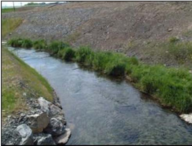
Newly created channel. The riparian grasses on the right bank have been transferred from the previous course of the now redundant original channel. The root structures stabilise the bank area while the grasses provide a degree of cover and shade and provide habitat for aquatic insects which form part of the food for fish.
