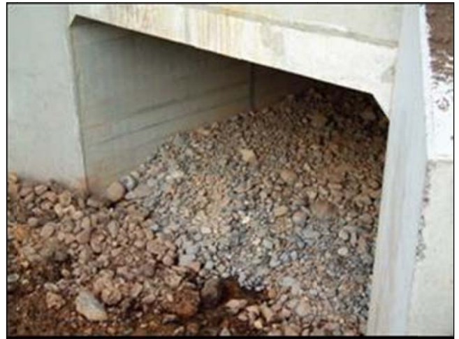
Off-line culvert at construction stage back filled with gravel. The size range and depth of fill required will be site specific.
