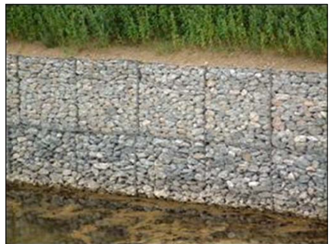
Visually unsightly stone filled gabion baskets.
