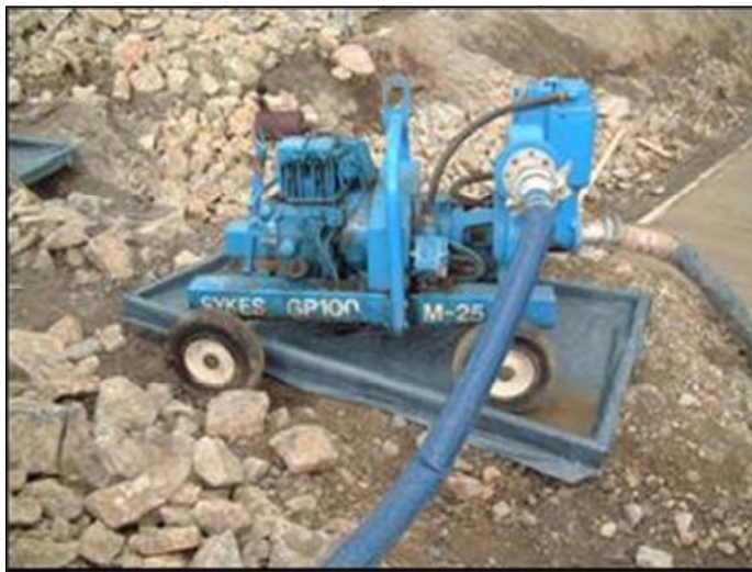
Poor work practice. The drip tray is undersized, constructed of too light a material, and accordingly overly flexible, easily damaged, and unlikely to retain oil residues.
