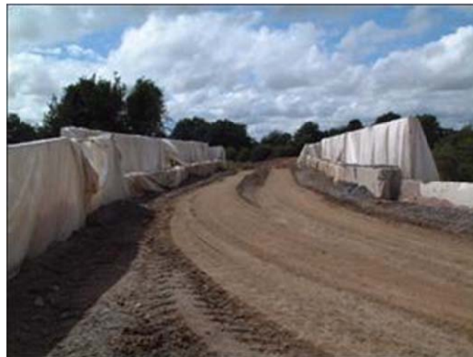
A crossing structure over a designated salmonid water. Note: terram covered fencing, reinforced concrete traffic barriers and fall back from the watercourse.
