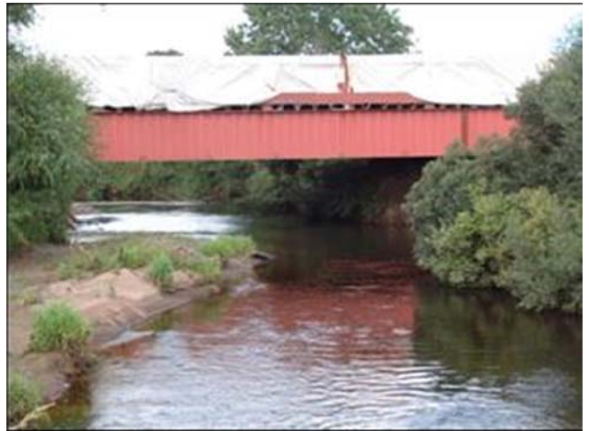
A clear span temporary crossing capable of carrying heavy axle loadings and long wheel base vehicles.
