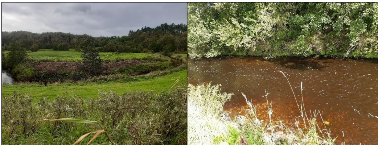
Plate 9. Examples of OPW drainage maintenance works, County River 2022.
