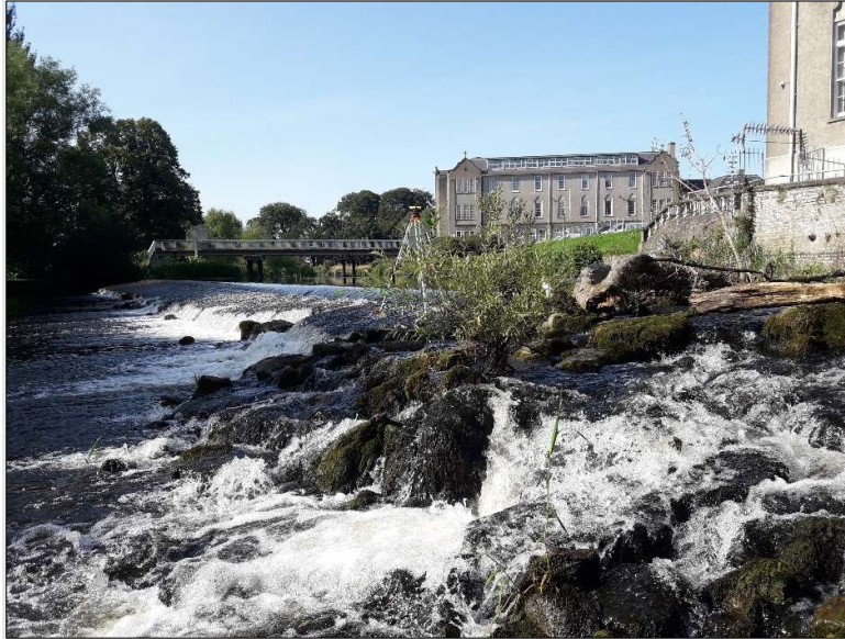
Figure 58. Broken section of weir (TS2).
