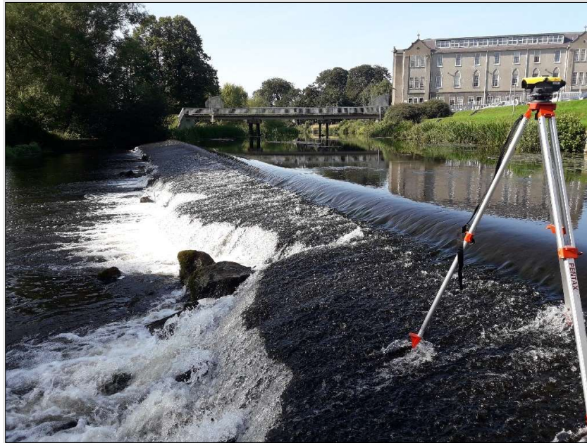
Figure 57. Weir face (TS1).
