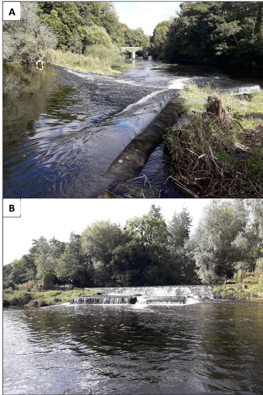
Figure 40. Fish passage option (TS1) from (A) upstream and (B) downstream.
