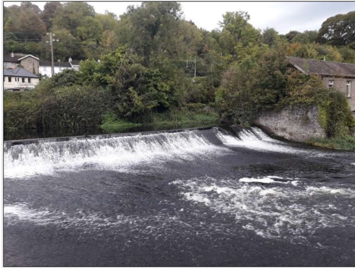
Figure 19. Weir face with crest lip (TS2).
