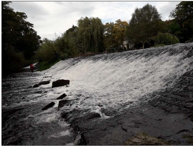
Figure 15. Weir face (TS4).
