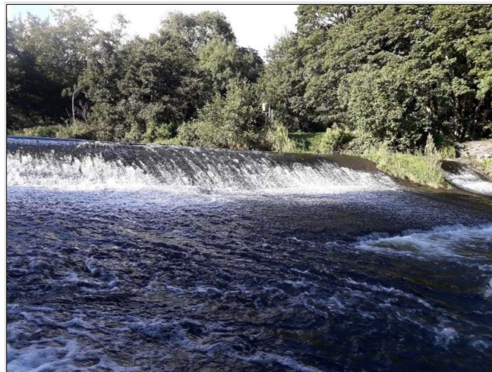
Figure 22. Weir face (TS1).
