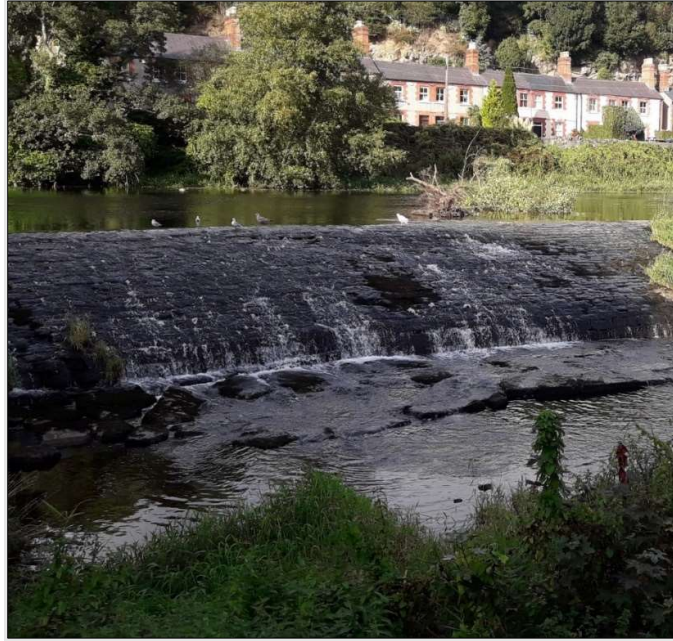
Figure 35. Weir face (TS3).
