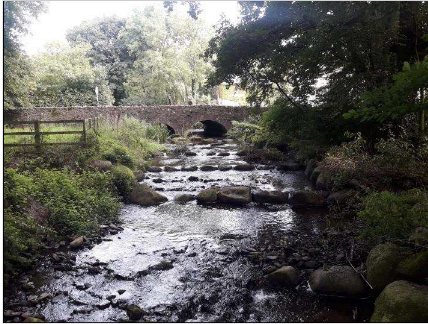
Figure 69. A full width pool and boulder rock ramp type fishway at Tuckmill Bridge, River Slaney, designed to mitigate the barrier impact of a bridge apron/culvert.
