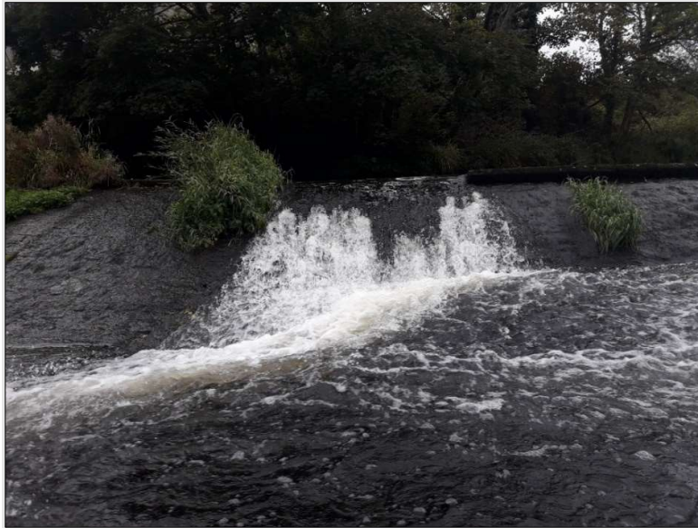
Figure 18. Weir face without crest lip (TS1).
