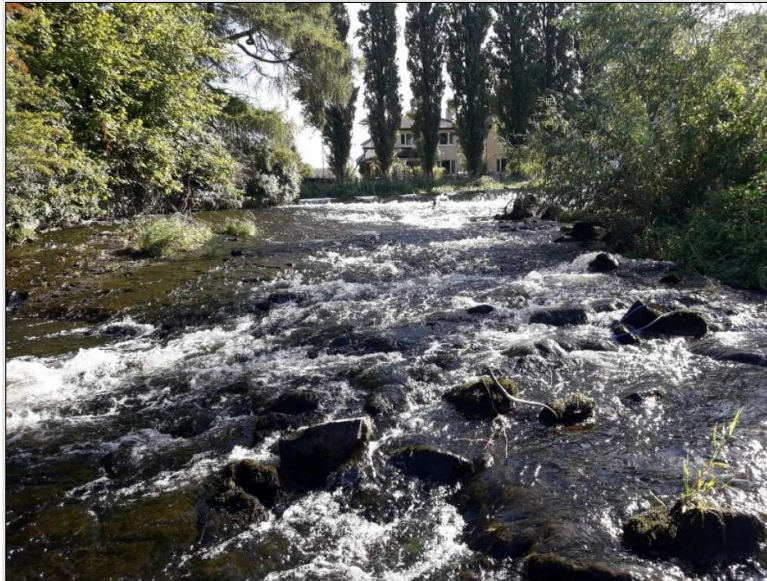
Figure 46. Weir face (TS3).
