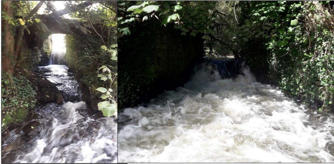
Figure 30. Sluices at Anna Liffey Weir.
