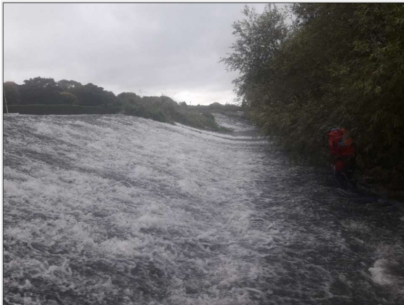
Figure 9. Sloping weir face (TS3).
