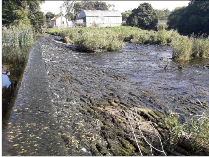
Figure 64. Weir face (TS4).
