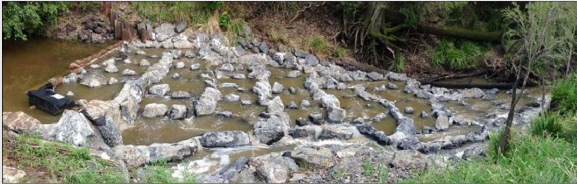
Figure 70. A full-width pool and boulder rock ramp fish pass designed to mitigate the impact of a weir on fish passage https://catchmentsolutions.com.au/portfolio/rock-ramp-fishway/
