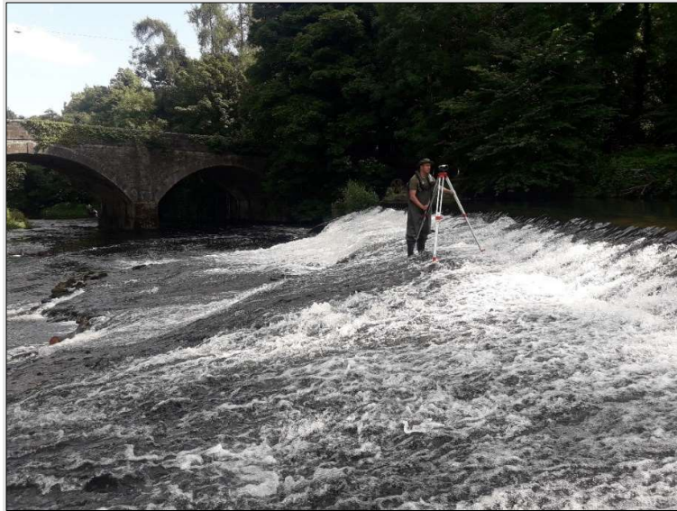
Figure 48. Weir face (TS1).
