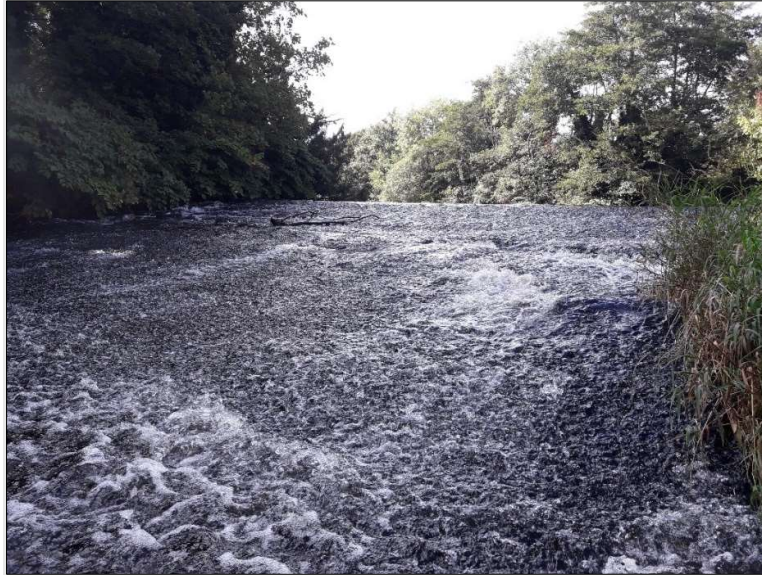
Figure 41. Weir face (TS2).
