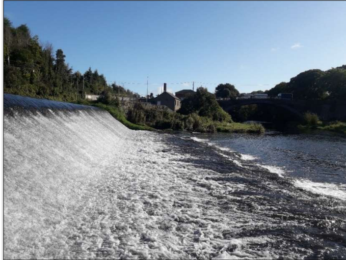
Figure 33. Weir face with rock sill (TS1).
