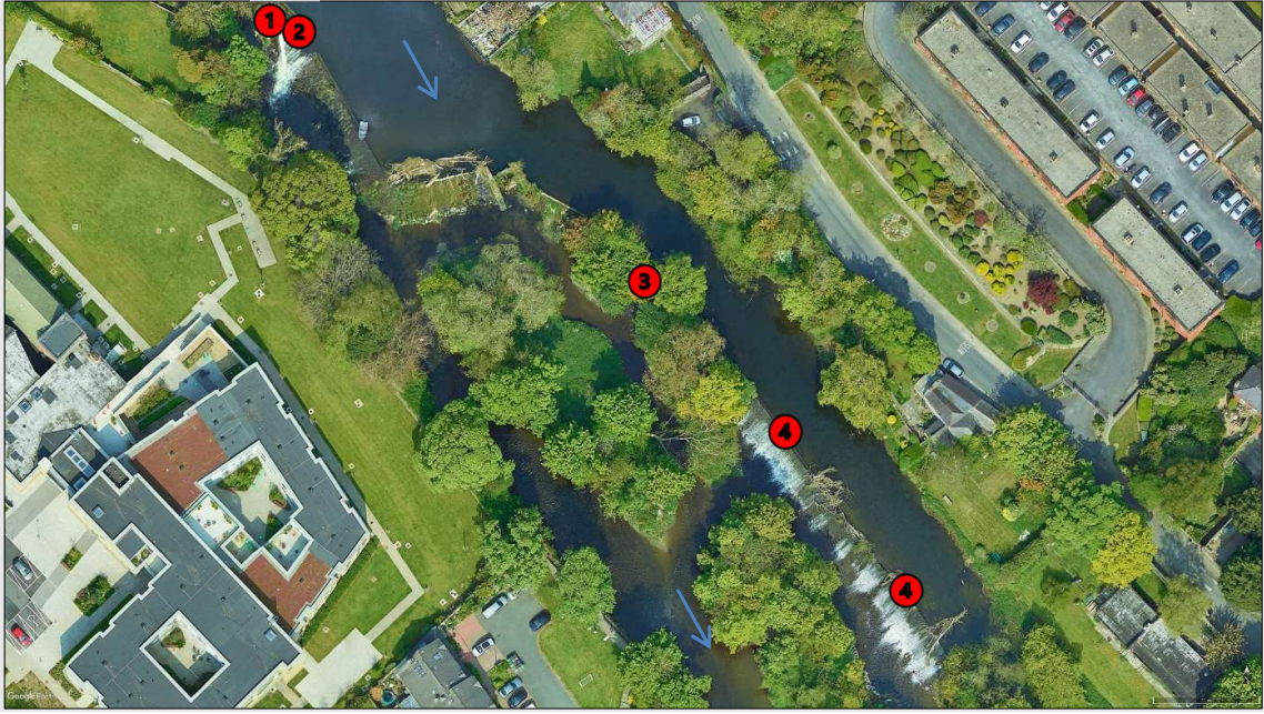
Figure 16. Google Earth ortho-image of Chapelizod Weir, April 2020. Blue arrows denote flow direction and red circles indicate transversal section number.
