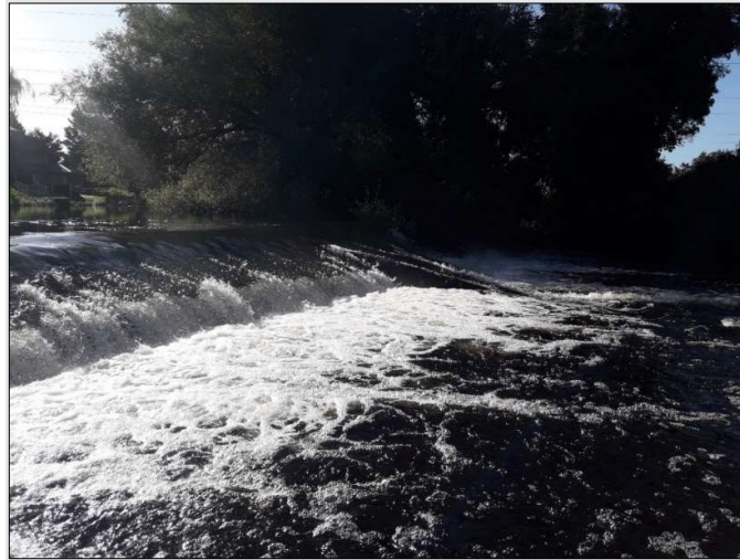
Figure 44. Weir face (TS1).
