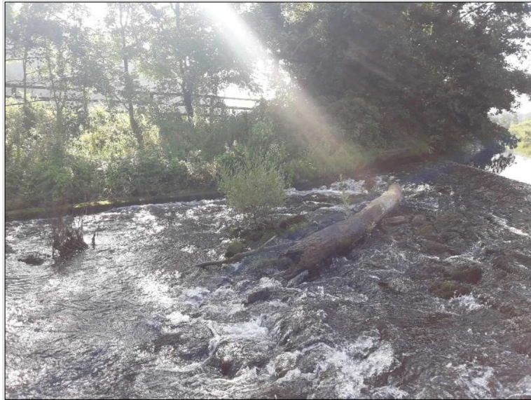
Figure 62. Weir face (TS2).
