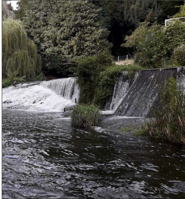
Figure 27. Vertical drop (TS1).
