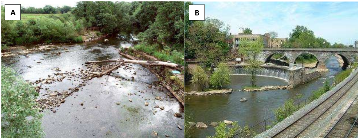
Figure 66. Photos of breached weirs: (A) Ballyclough Weir in the Mulkear River, Co. Limerick, and (B) Kent Dam in the Cuyahoga River, Ohio, USA (breach in far right of image).
