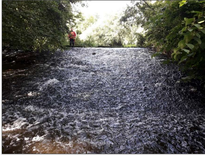
Figure 42. Weir face (TS3).
