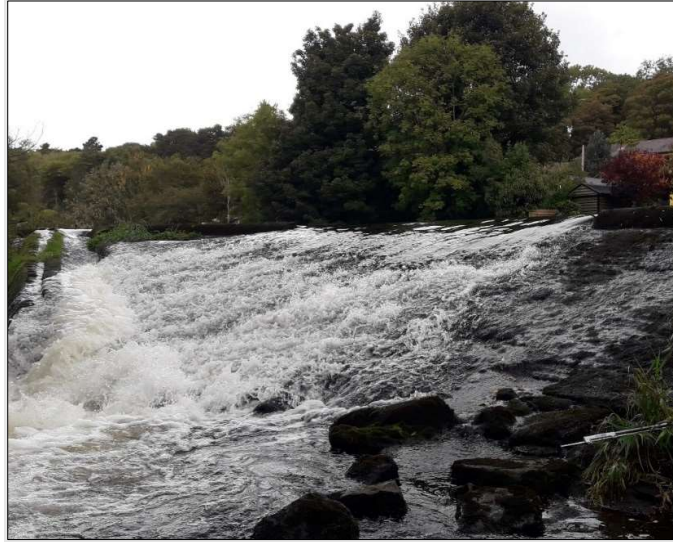
Figure 13. Breach into TS1 by TS2.
