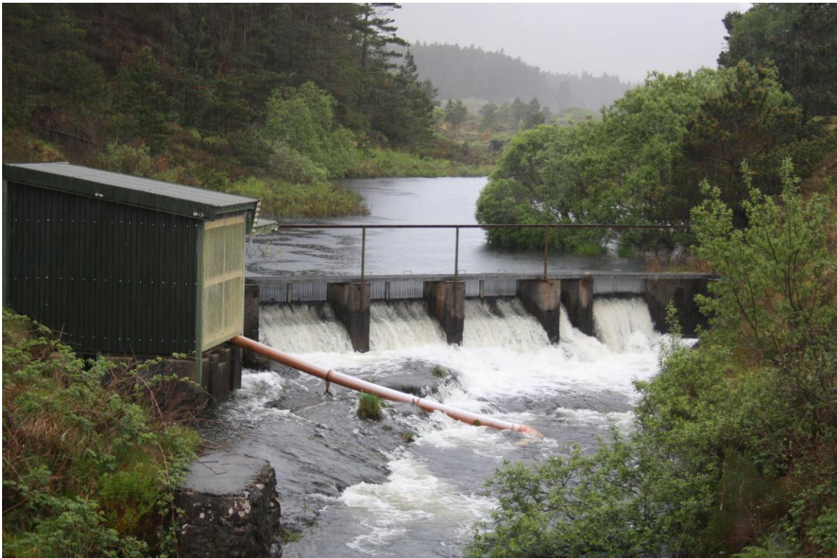
Figure 3 Wolf-trap located along the outflow from Tawnyard Lough captures downstream migrating smolts and kelts.
